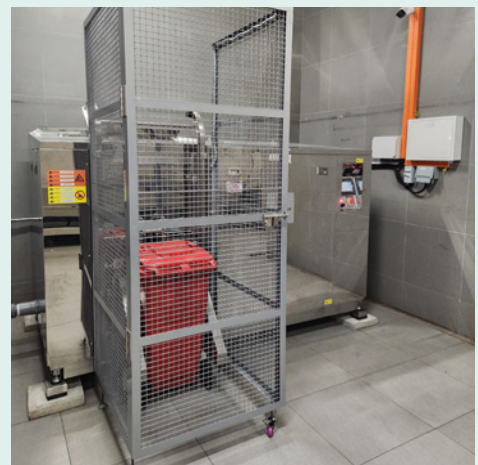
Food waste biodigester installed at Funan which commenced its pilot in late 2022
