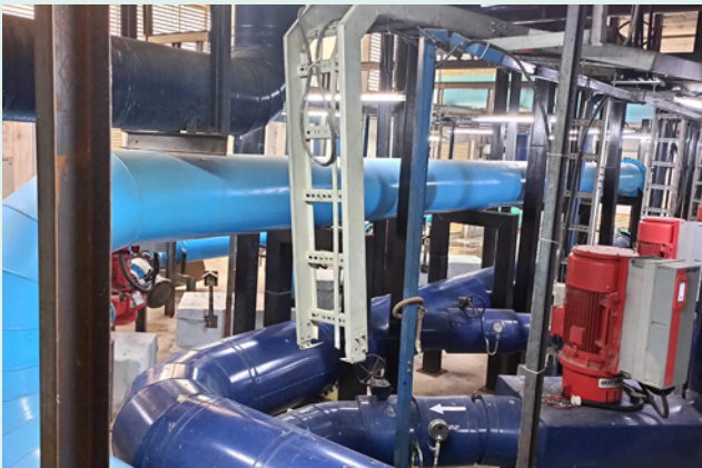
Chiller plant rooms with interconnecting chilled water header pipes
